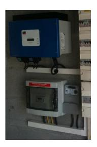
The meter can be installed on the wall or on an electrical panel or inside a case.
